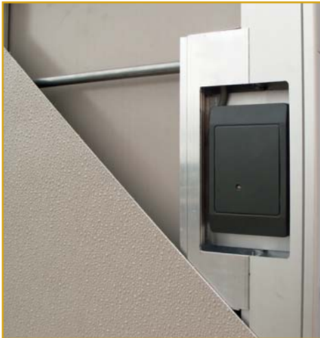
Cut-away reveals how door was prepped for card reader location
