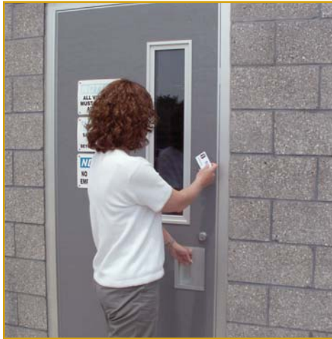
Wave card in front of internal reader to release lock mechanism
